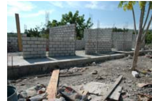
Classroom walls being built
