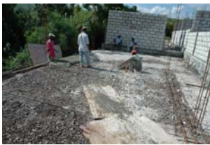
Getting ready for concrete one bucket at a time.
